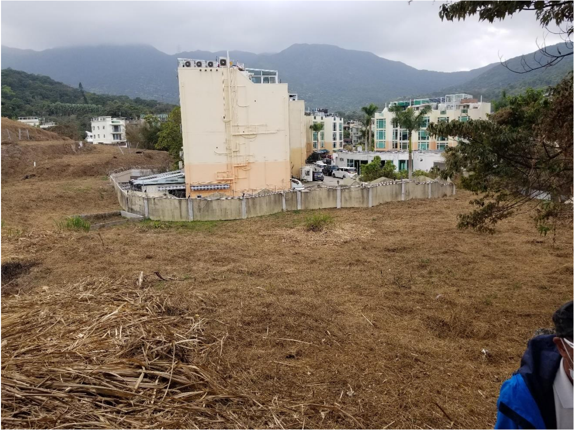
Photo C Close View of the Northern End of the Site, Looking West
